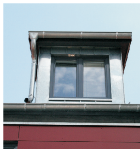
Dormer and bay insulation
