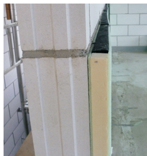
Ceiling/Internal wall insulation
