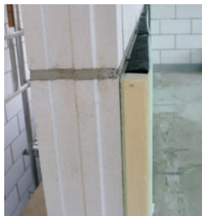
Ceiling/Internal wall insulation
