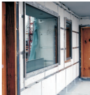
Façade insulation - B1/B2 Fire protection façade with approval
